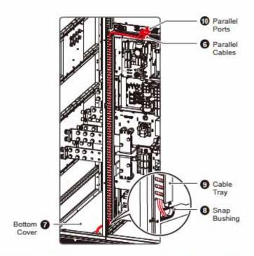
(Figure 5-39: Bottom Entry & Location of Parallel Cables, Bottom Cover, Snap Bushing, Cable Tray and Parallel Ports)
